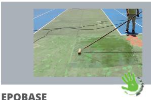
EPOBASE is a solvent-free epoxy resin based twocomponent primer, that is ideal as primer for polyurethane and epoxy resin systems. The product is generally used on highly porous or low porous cement decks, both as primer and quartz binder for synthetic mortars.
